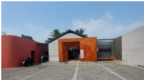
Gambar 2.. Fasad Manca Eatery Cafe Sumber: Data Pribadi
