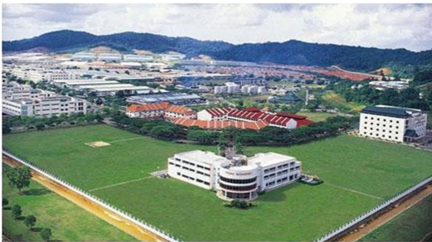
Figure 3. Showing the Batamindo Industrial Estate, which is Very Relevant to the Madani City Landscape
